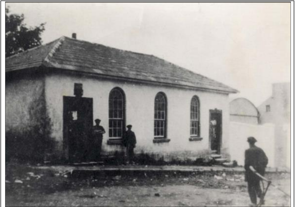
Historic Sites: Kinvara courthouse after the roof had been replaced Source: https://kava.ie/history-of-courthouse/
